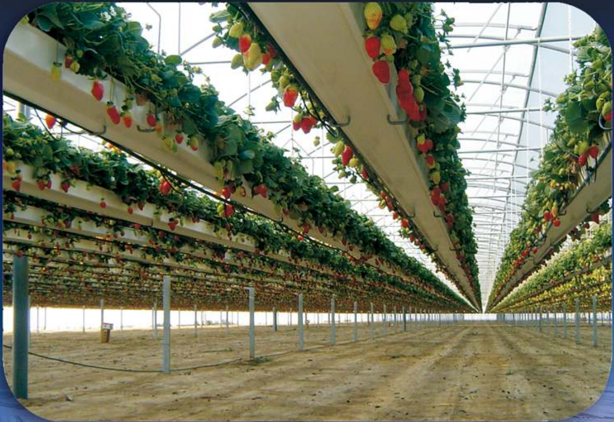
PVC Drainage Canal
